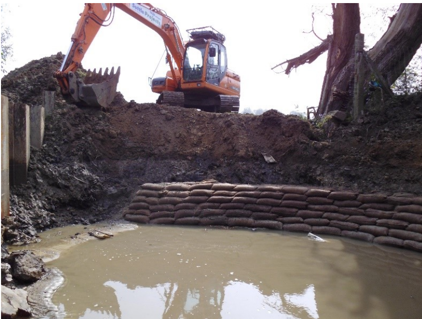
Figure 3: Bagwork with cofferdam
