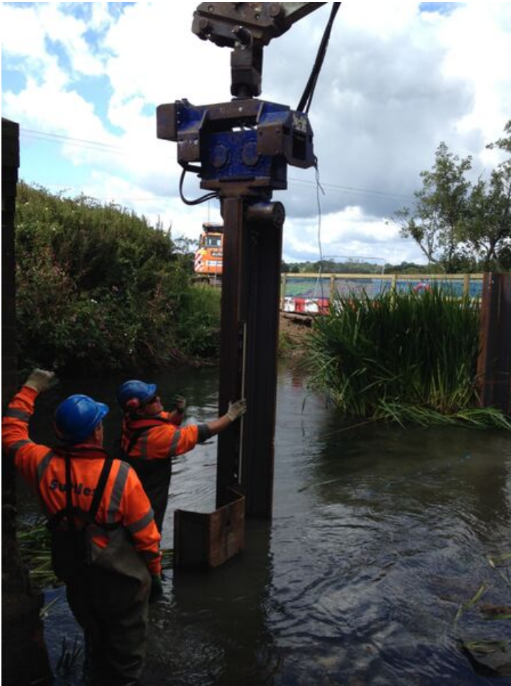
Figure 2: Cofferdam installation
