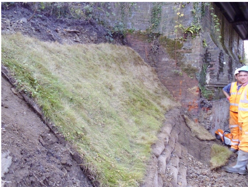
Figure 1: Construction of downstream banks
